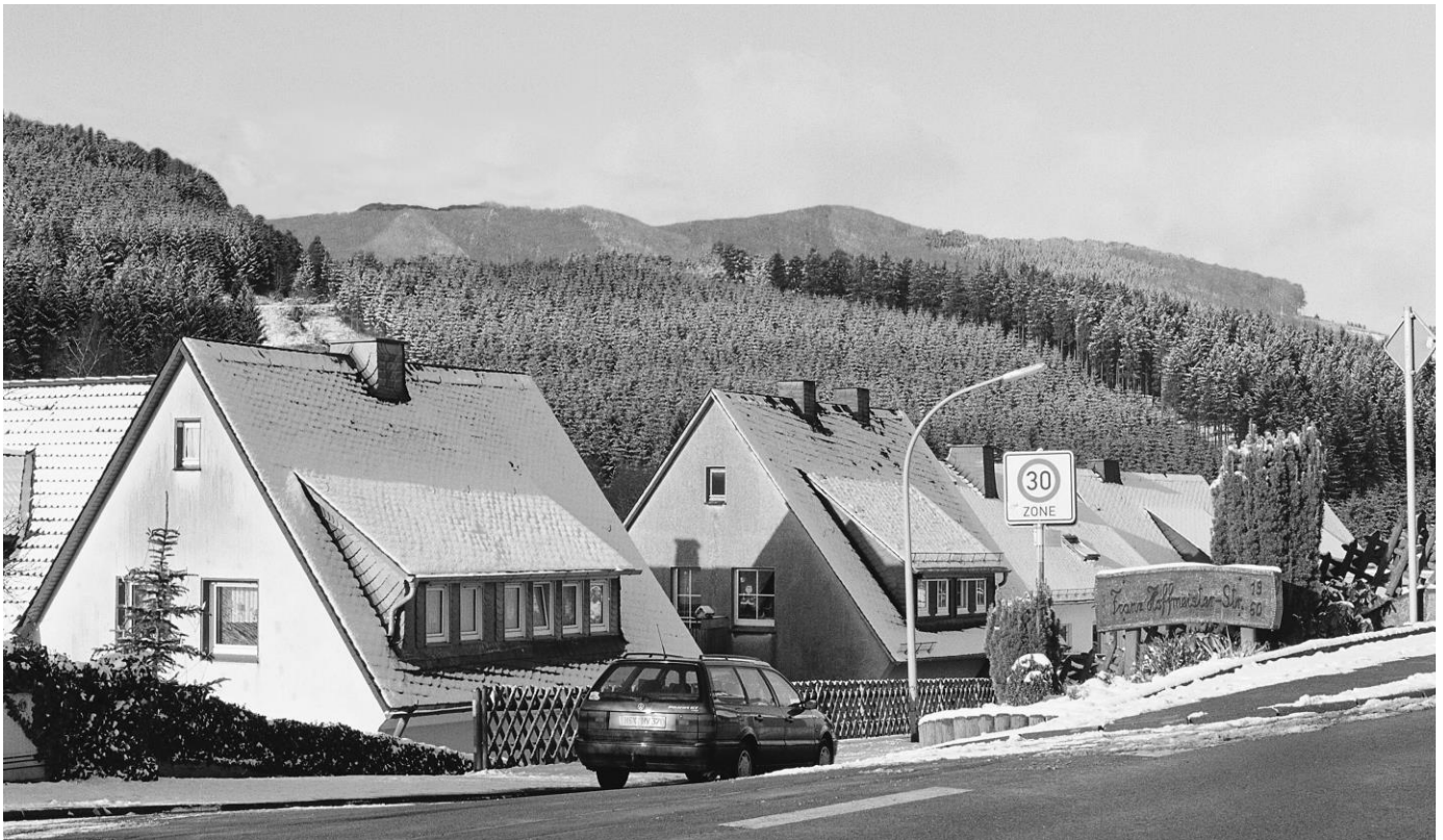
Figure 12. Refilled final stage of opencast
